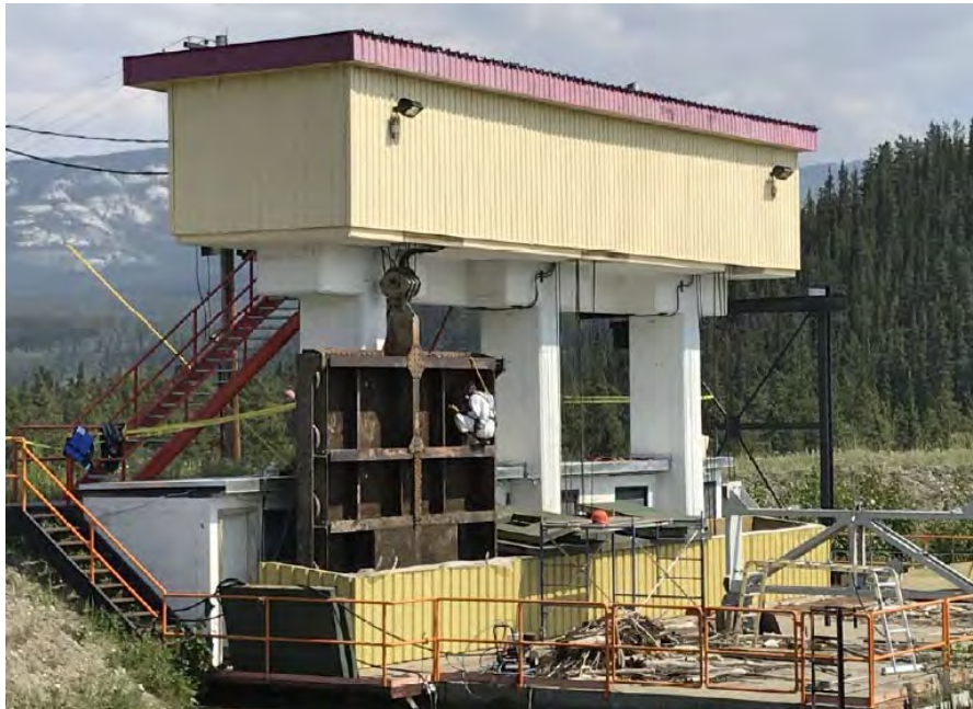
Photograph 1 - WH1 Headgate Inspection Position
