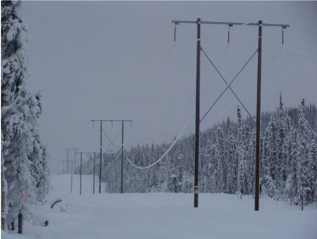
Figure 4.1 – Extreme Rime Ice on L174 (2011)
