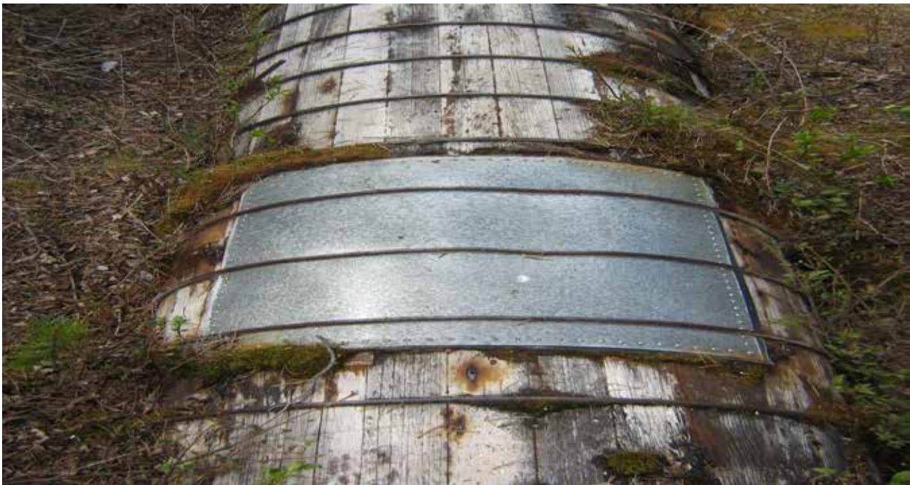
Figure 4 - Photo of Patch Repairing a Leak
