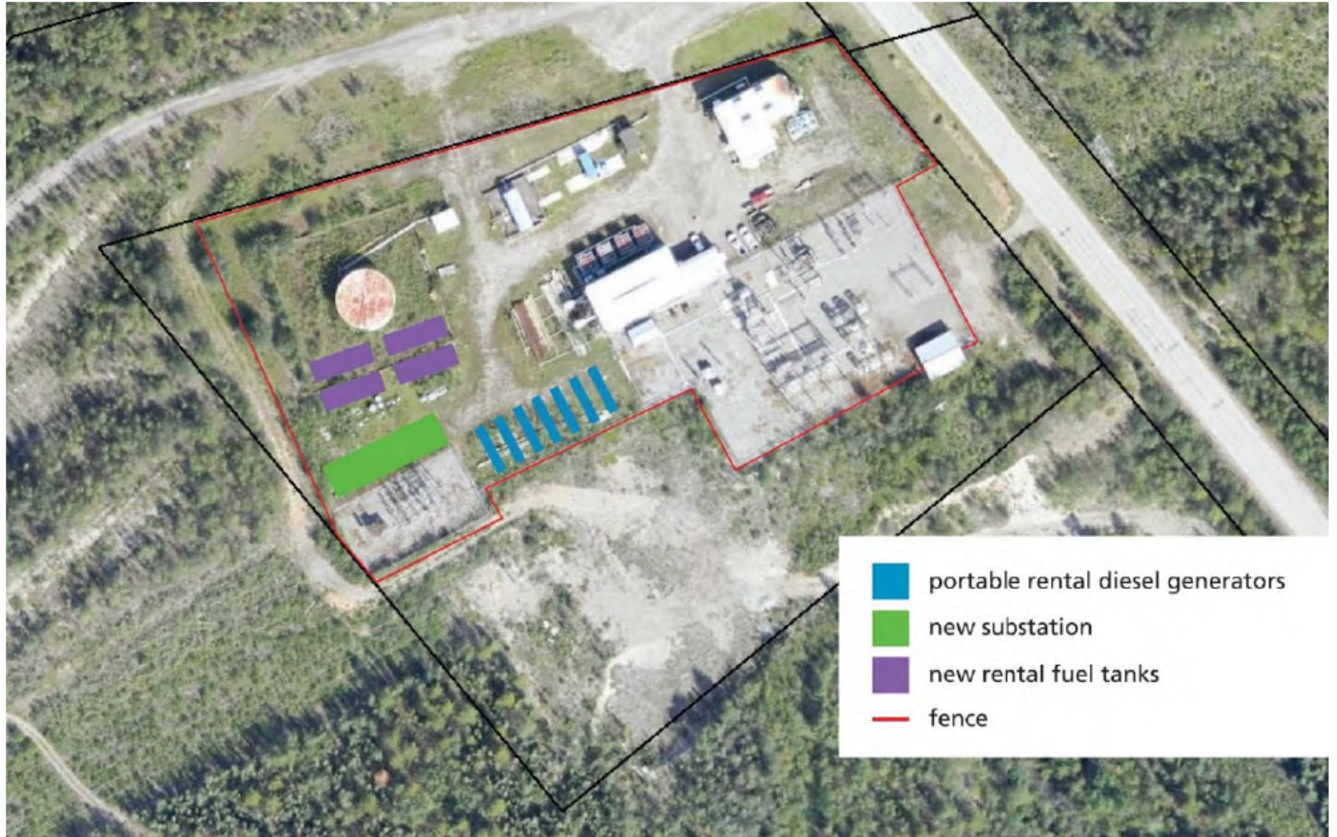
Figure 2: Faro Generating Station Site Overview
