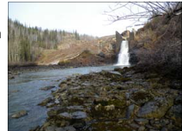
Wareham Lake spillway
