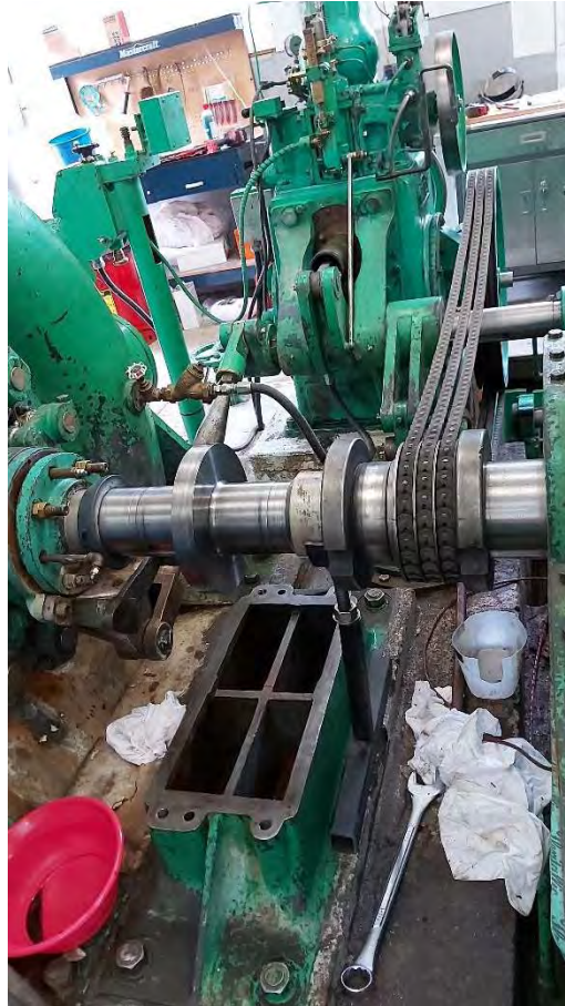
Figure 11: Gilkes Governor Belt Drive (Speed Indication)
