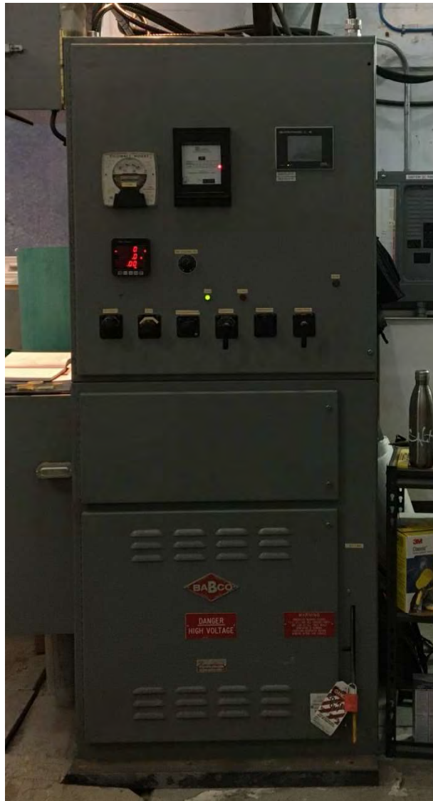
Figure 19: P&C and SWGR Panel
