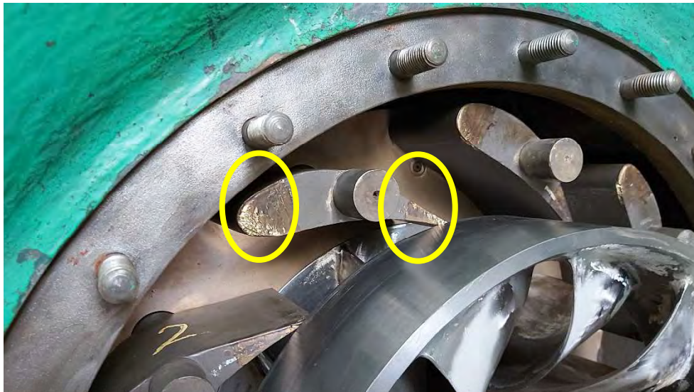
Figure 4: Wicket Gate Damage
