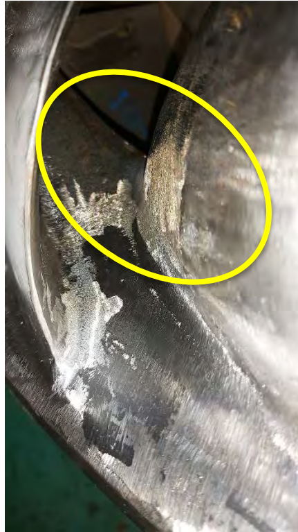
Figure 2: Runner Suction Side Cavitation (expansion too severe)
