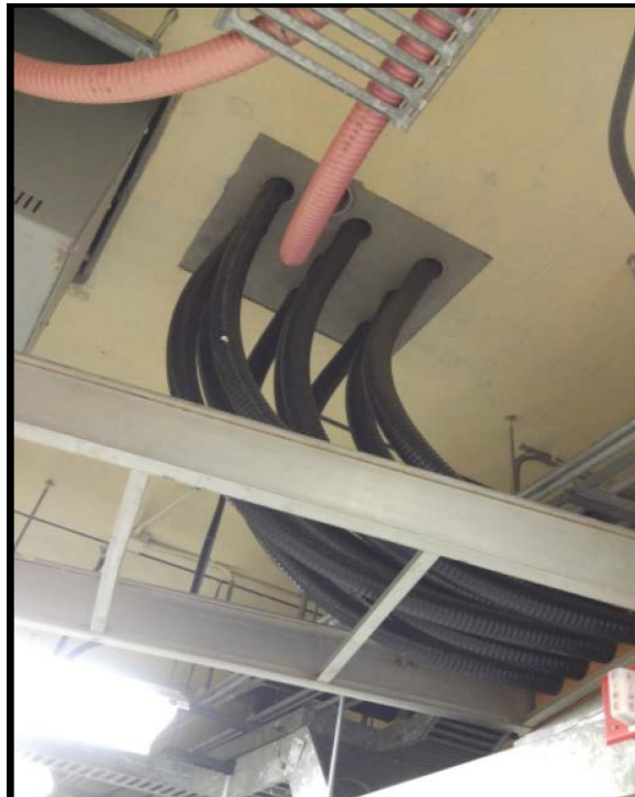
Figure 5-2: Generator Lead Arrangement
