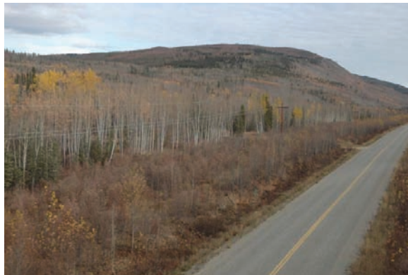
Figure 6. Aerial view of ROW showing ground and edge conditions, note tall brush on ROW requiring mowing (Line L 174).
