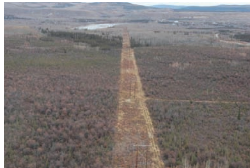
Figure 8. Typical aerial view of ROW showing ground and edge conditions, (Line L 173A).
