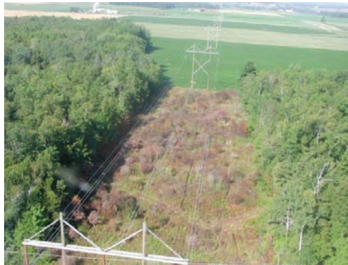
Figure 19. Example of good brush control through the use of herbicides (Wisconsin, U.S.).
